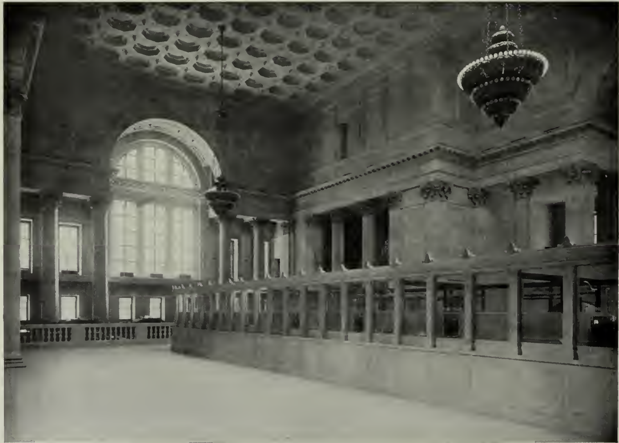
INTERIOR VIEWS, NATIONAL CITY BANK, NEW YORK CITY.
